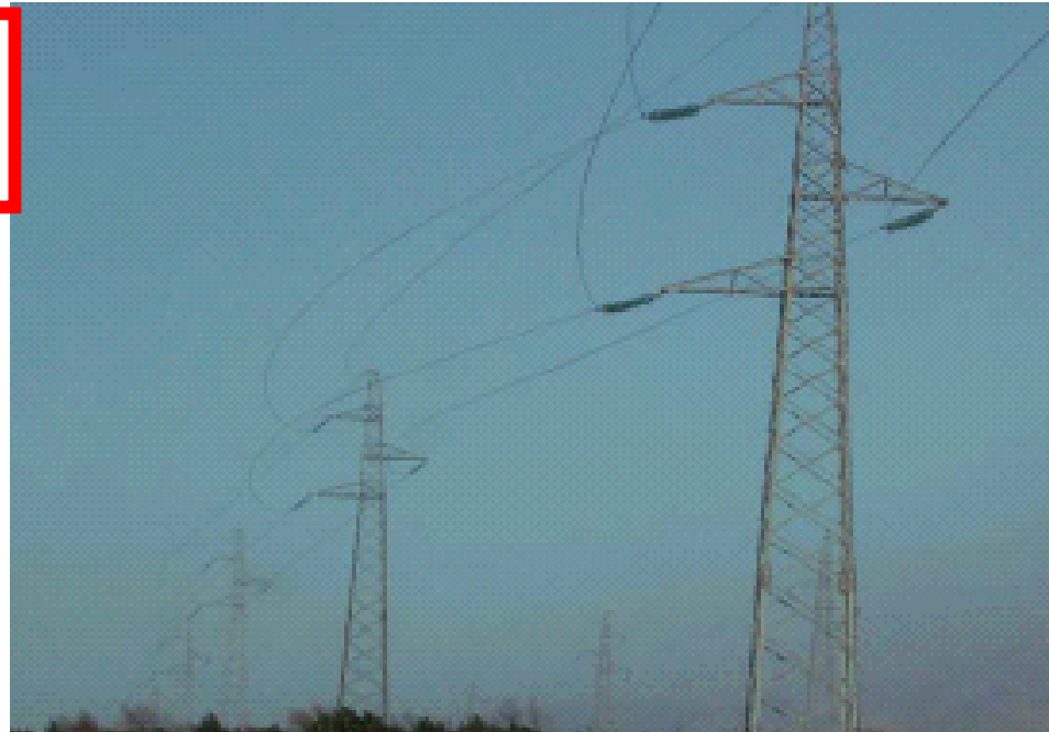
Figure 2.17 Conductor blow out during 'Bora' Wind Storm in Croatia- Jan 2003 (Photograph courtesy F Jaki)
