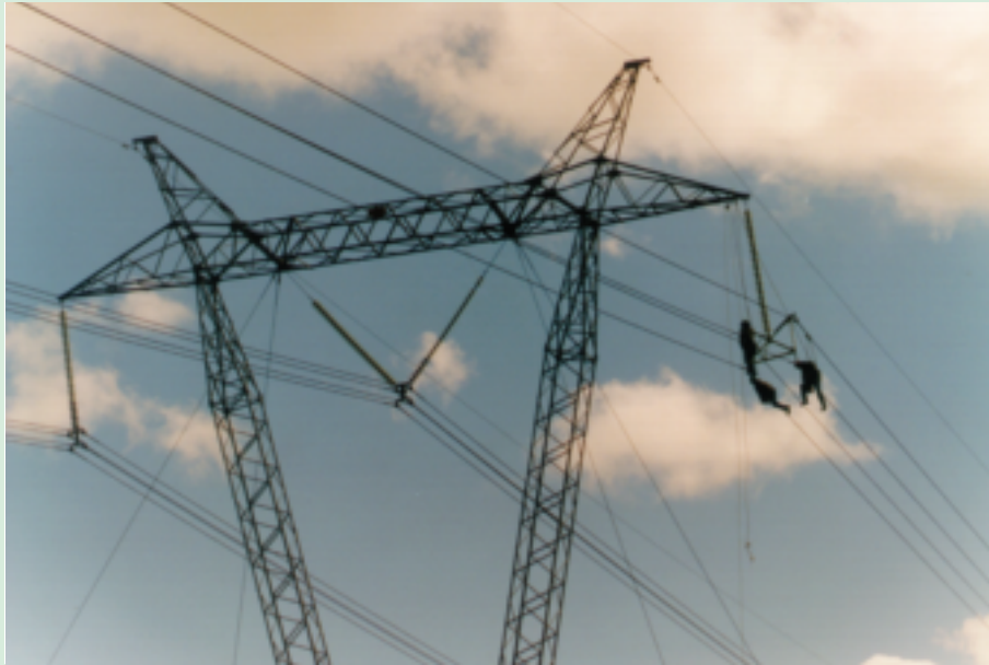
Fig. 2: Expanded bundle on right hand phase under construction [10]
